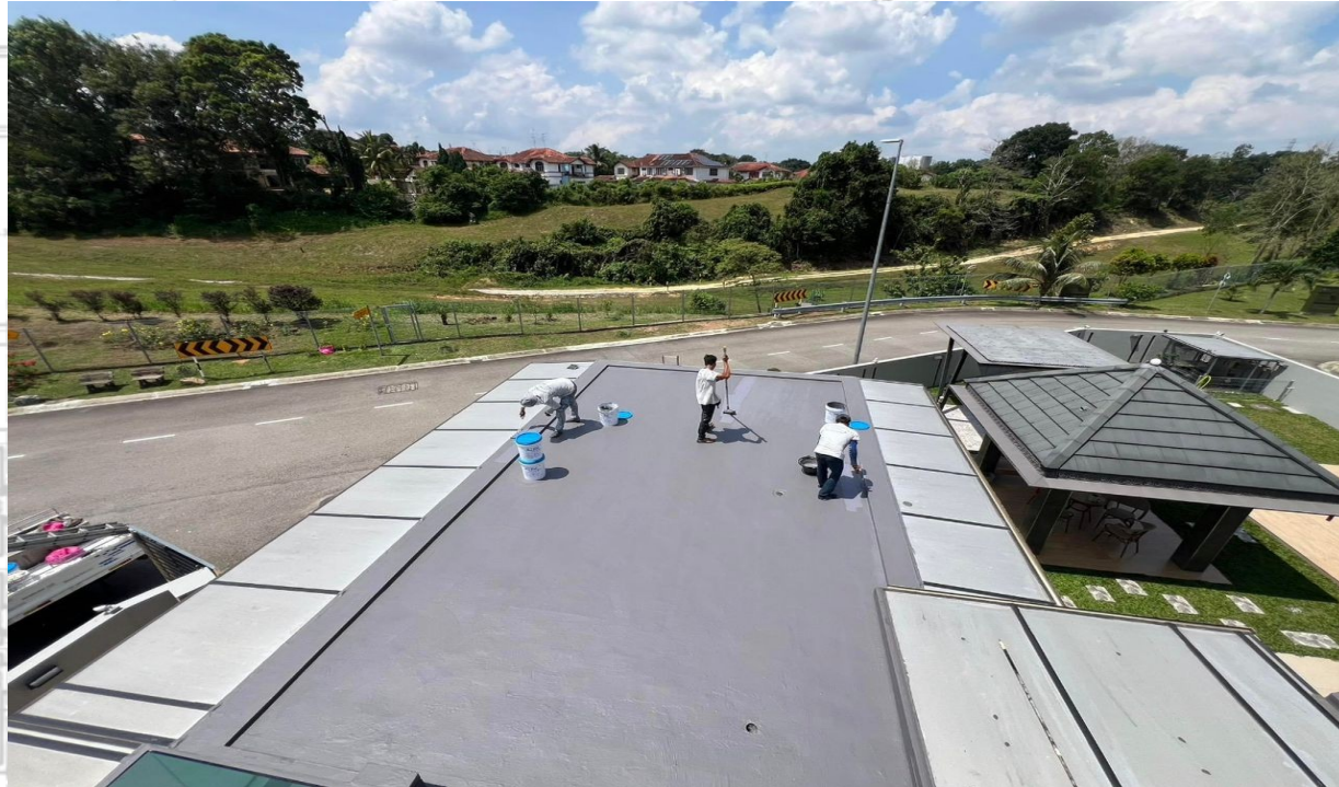
Water Proofing work @ Balik Pulau, Penang
